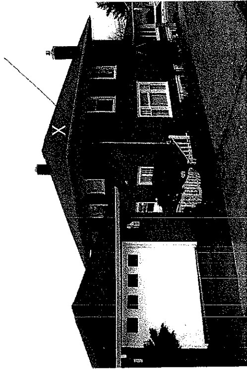
Unused center roof chimney; removal proposed. Site (X) for placement of south-facing vented skylight.
