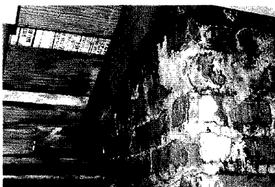
In attic, unused chimney moisture and mold damage.
