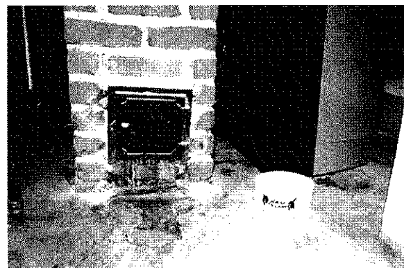
In basement, water drainage at base of unused chimney
